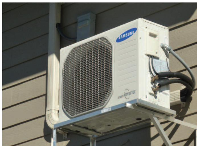
*The condenser unit for a mini-split heat pump system is usually mounted on an exterior wall. Photograph by Gary Cziko*
