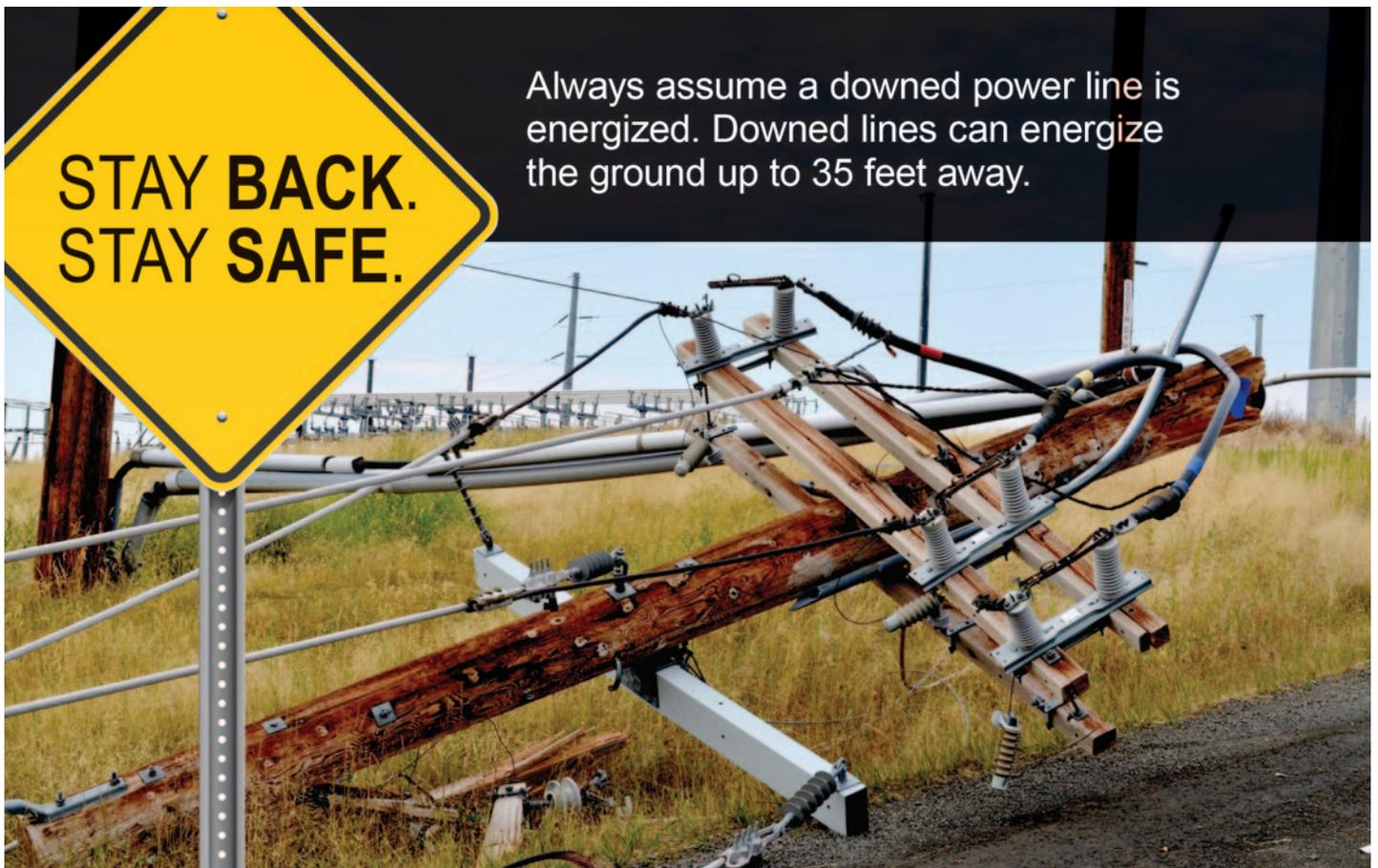
Always assume a downed power line is energized. Downed lines can energize the ground up to 35 feet away.
